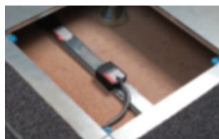
Busbar Electrak
